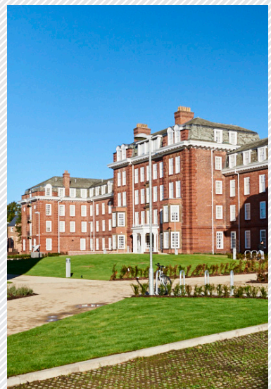
Neville House, Sheraton Park, Durham
